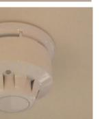
If the detector starts making a short beep/chirp sound, this is an indication that the backup battery should be replaced. In order for the detectors to work properly it is essential that batteries are changed when required.
