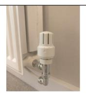
The desired temperature in each room can be set by adjusting the TRV valve on the individual radiators.
