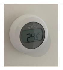
The thermostat for your heating system primarily operates by sensing the air temperature of the surrounding room. The thermostat will then regulate the system to reach your desired temperature setting, pausing once this temperature has been met. The thermostat can be found in the living room of the apartment.
