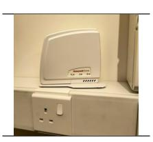
Honeywell is a device found in the Utility cupboard that allows you to program your heating to come on at a specific time using the app on your smart phone.
