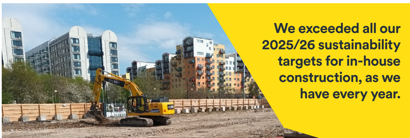
Hybrid excavator at Greenwich Peninsula
